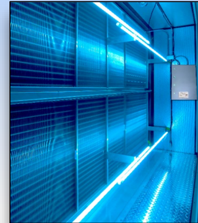
HVAC Coil/Surface Cleaning
