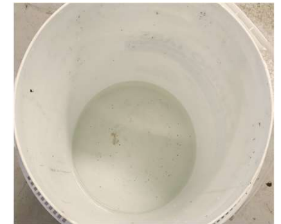
Condenser water before start-up (looks clean)
