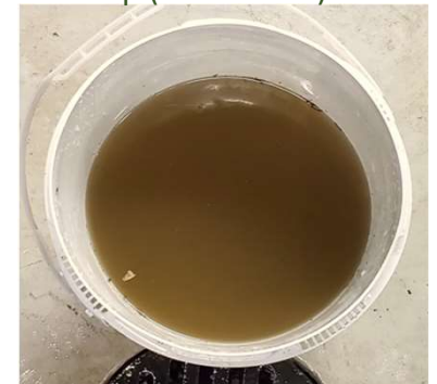
Particles removed from condenser water in 1 week
